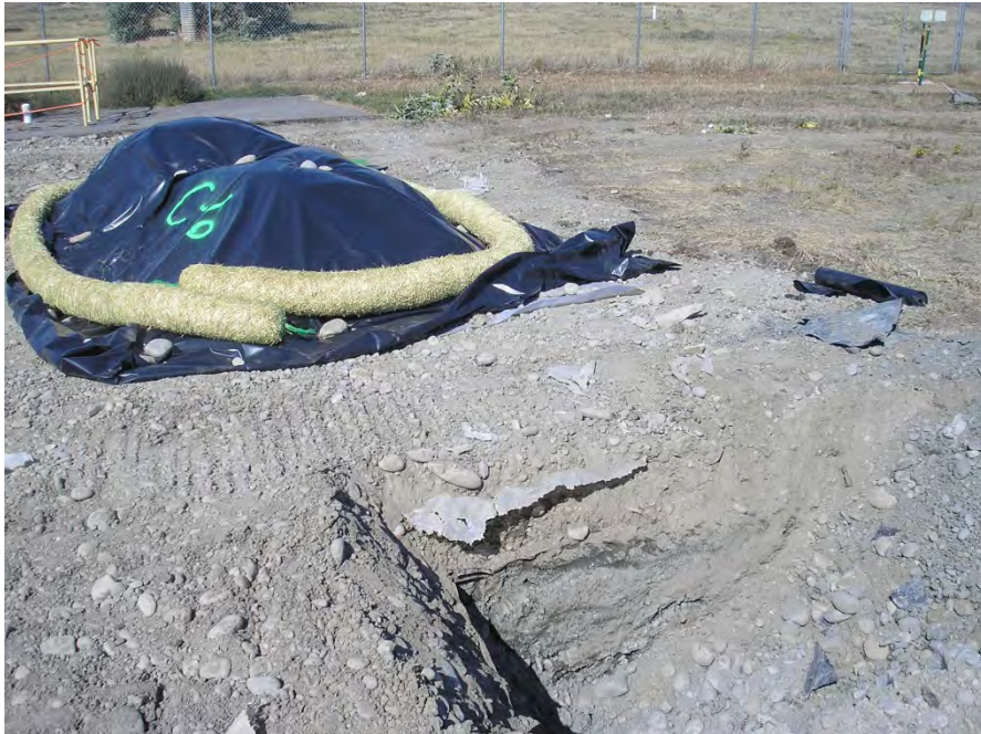
Pond C – Test Pit C-6 in northwest corner.
