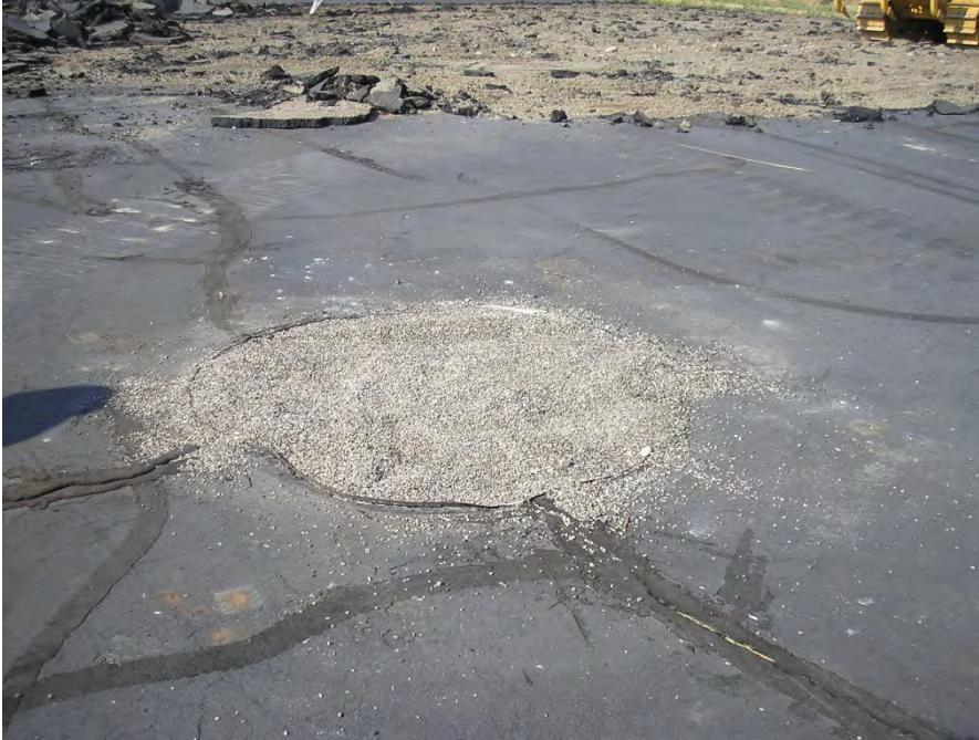
Location of abandoned monitoring well M-19
