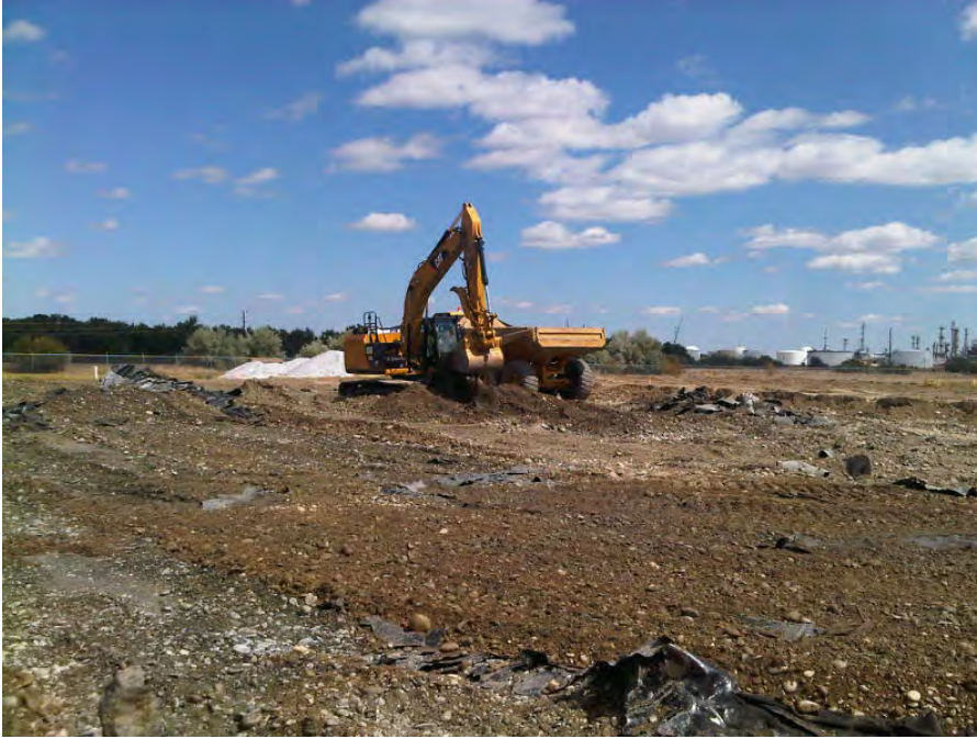
Loading overburden into dump truck for transport to stockpile. Facing northeast.
