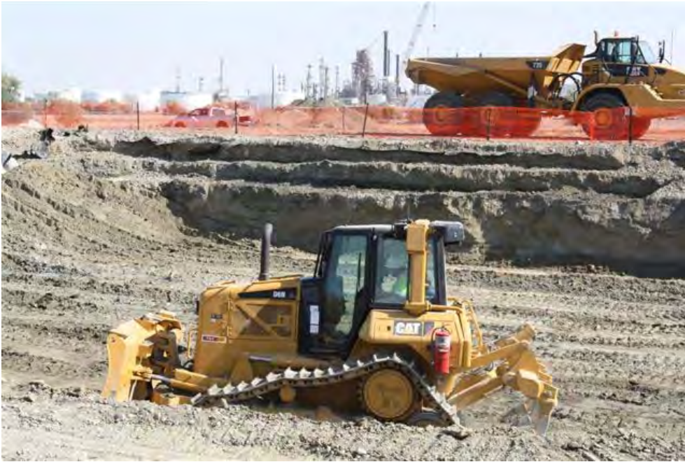
Pond C – Excavation in process. Facing southeast.
