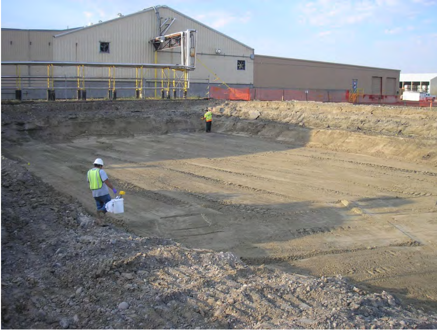
Pond A – Preparing for sample collection following excavation. Facing southwest.
