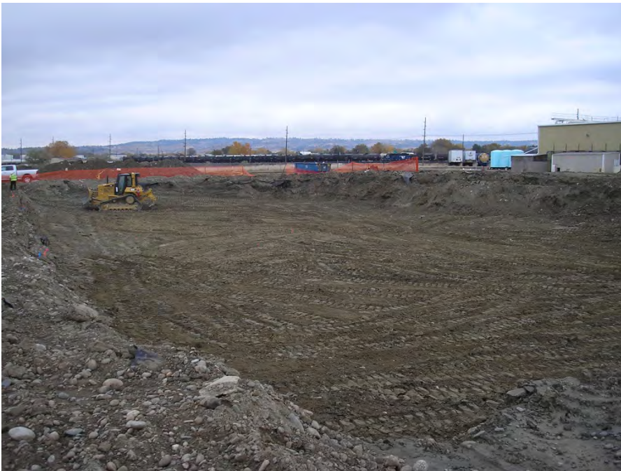
Pond C – Extent following excavation. Facing southeast.
