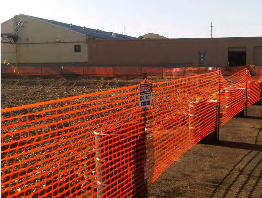
Fencing and signage around Pond B. Facing south.
