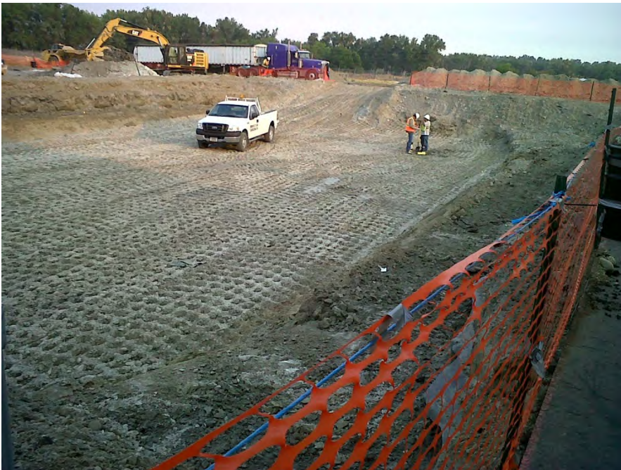
Pond A – Compaction testing during backfill activities. Facing north.
