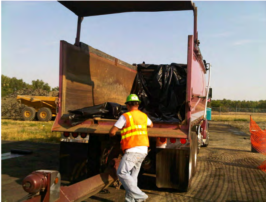
Waste disposal truck bed – lining prior to loading.
