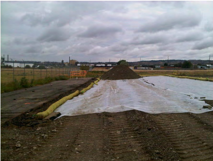
Stockpile. Facing east.
