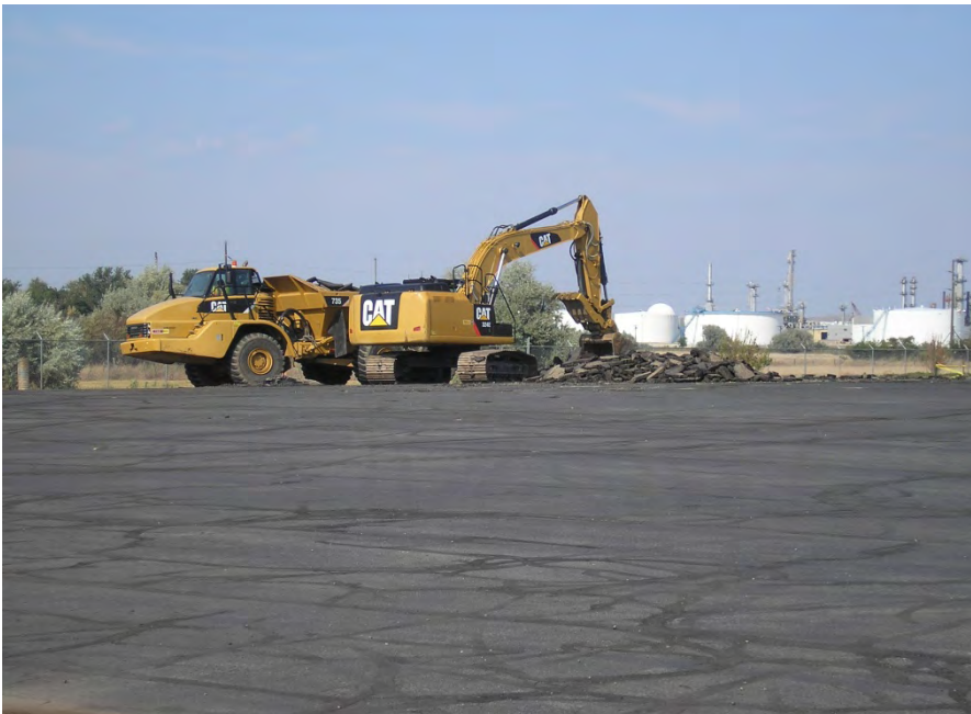
Removal of asphalt cover over surface impoundments. Facing Northeast.
