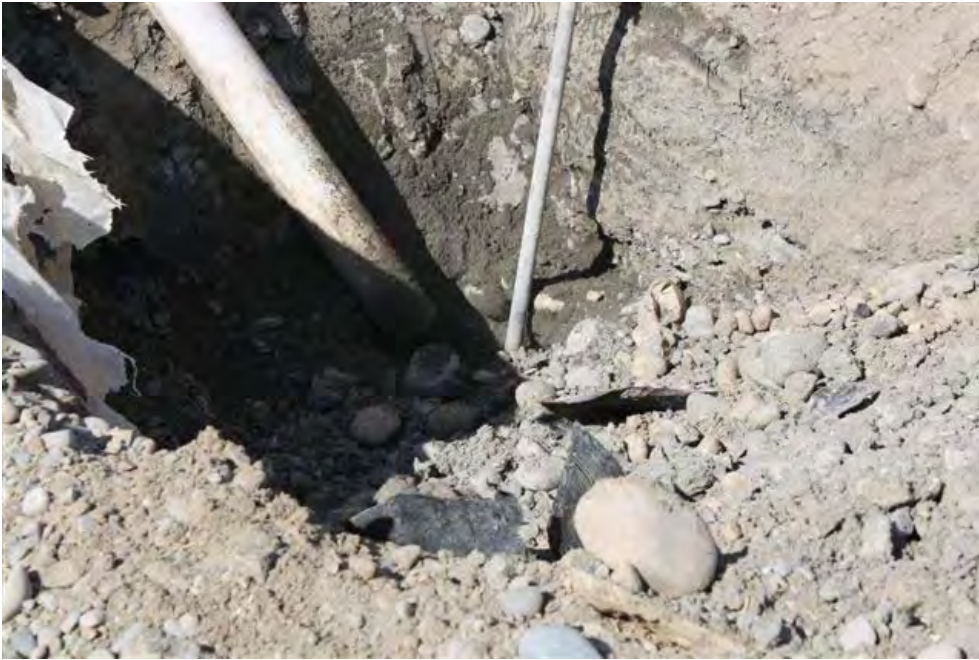
Pond C – Potholing to locate depth of bottom liner.
