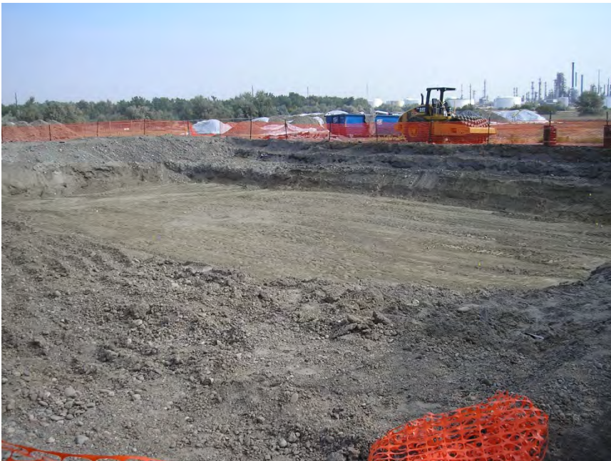
Pond B – Extent following excavation. Facing northeast.
